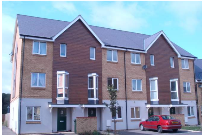
New houses, Northfleet
